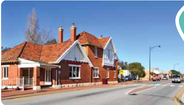
Coopers Mill & George Street
