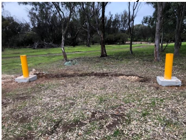
Figure 1: Example of completed bores
