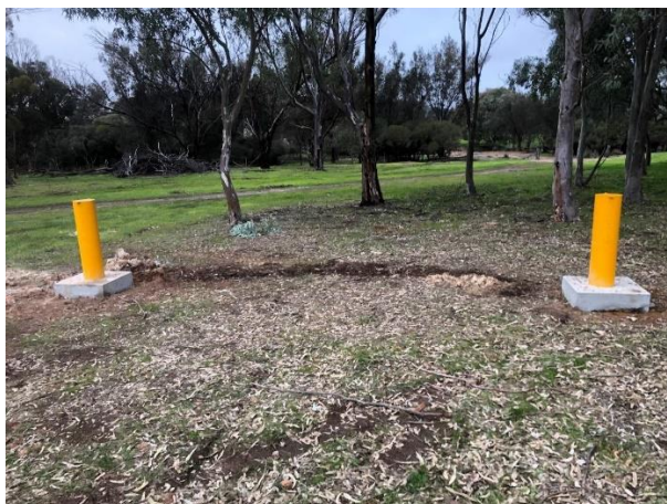
Figure 1: Example of completed bores
