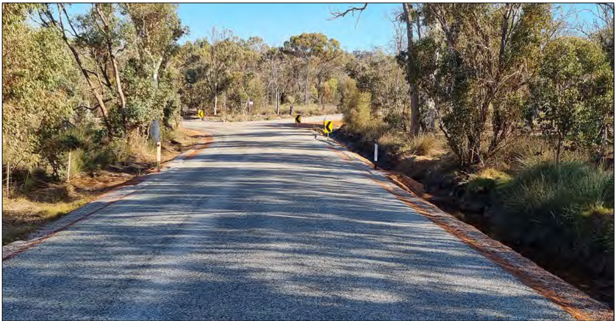
Moramocking Road after completed works
