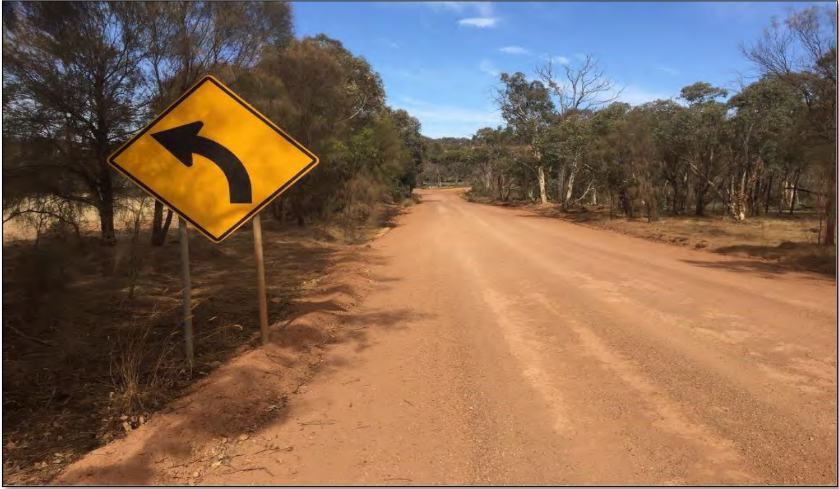
Moramocking Road prior to the works
