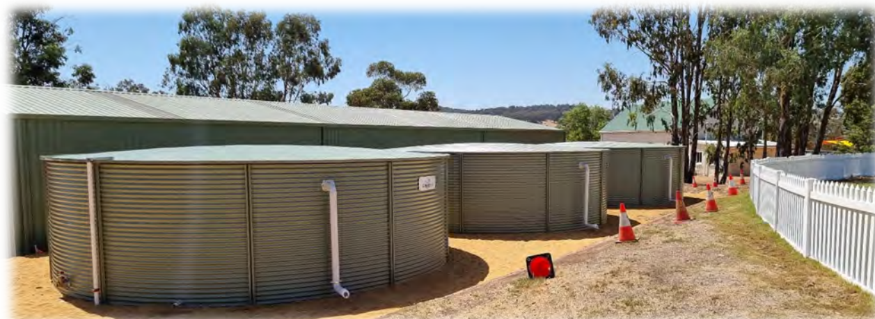
Collecting rain water run off from the machinery shed to re use at the public toilets
