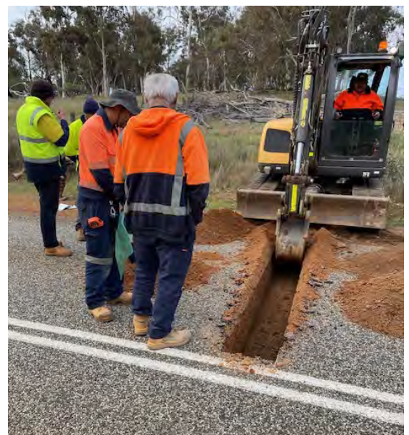
Test holes completed along North Bannister Wandering Road for WSFN.
