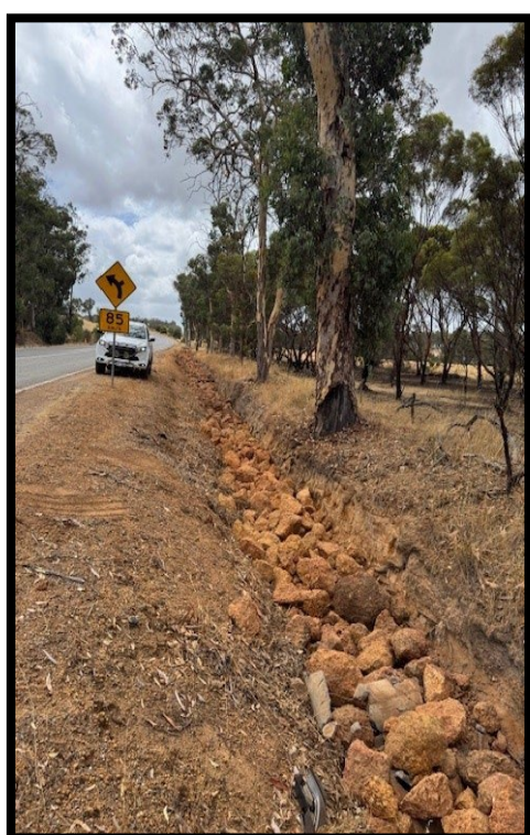
Wheatbelt Secondary Freight Network – Subsoil Drains
