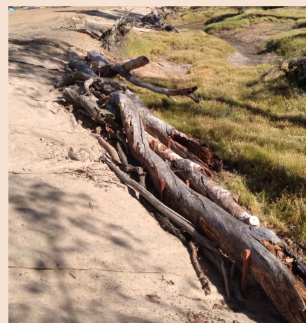
Example of using logs on riverbanks – Pumphreys Bridge
